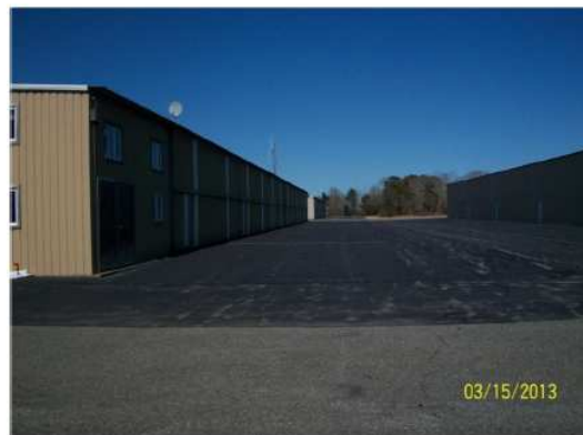
Figure 3: Rear View of Hangar B
