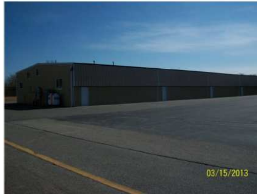
Figure 2: Front/Side View of Hangar D
