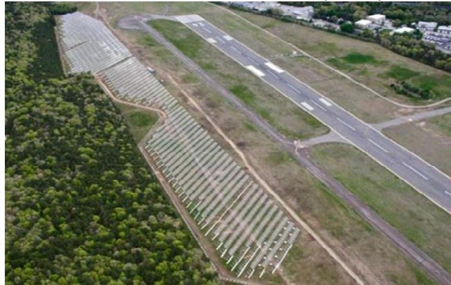
Figure 5.19 Solar Panels at Barnstable Municipal Airport
