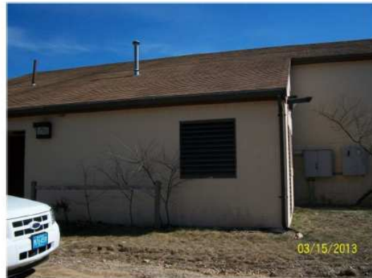
Figure 2: Front View WWTP
