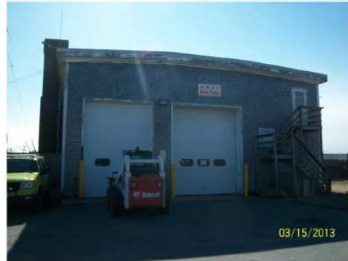
Figure 4: Landside View of ARFF/SRE Building
