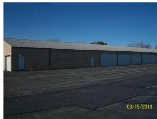
Figure 3: Rear View of Hangar E
