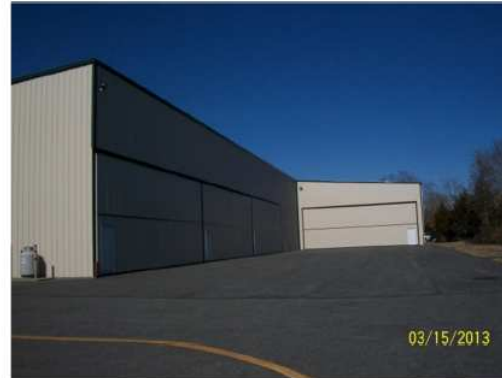
Figure 4: Rear View of Hangar H
