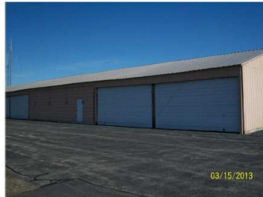
Figure 2: Front View of Hangar F
