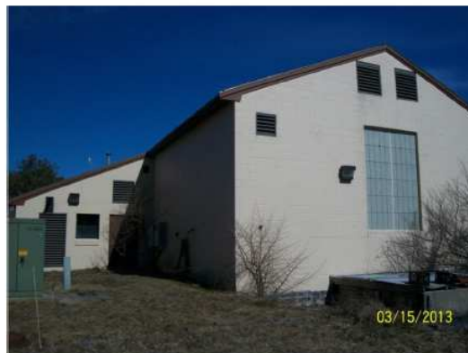
Figure 3: Side View WWTP
