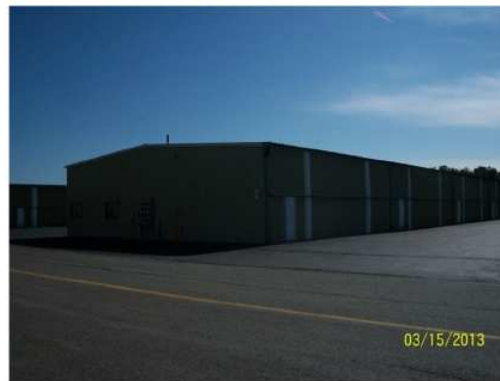
Figure 2: Overall view, Hangar A
