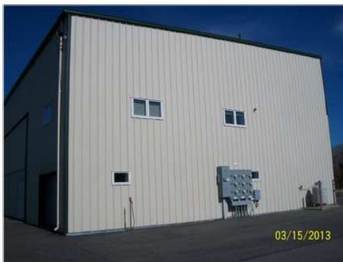
Figure 3: Side View of Hangar H
