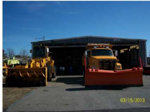
Figure 2: Front View of Hadley Hangar
