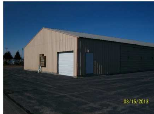
Figure 2: Rear/Side View of Hangar E
