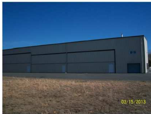
Figure 2: Front View of Hangar H
