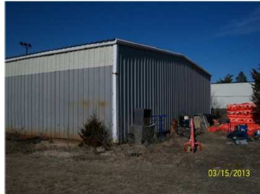
Figure 4: Rear/Side View of Hadley Hangar
