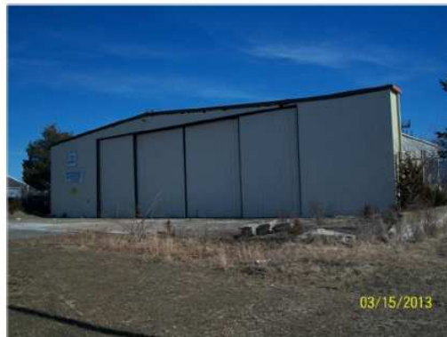
Figure 2: Front View of Duchess Hangar
