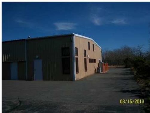
Figure 3: Front/Side View of Hangar D
