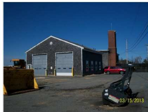
Figure 2: Airside View of ARFF/SRE Building
