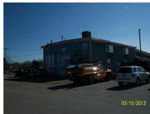
Figure 3: Landside View of ARFF/SRE Building
