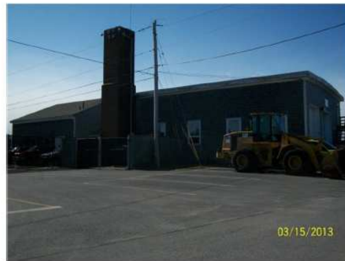
Figure 5: Landside View of ARFF/SRE Building
