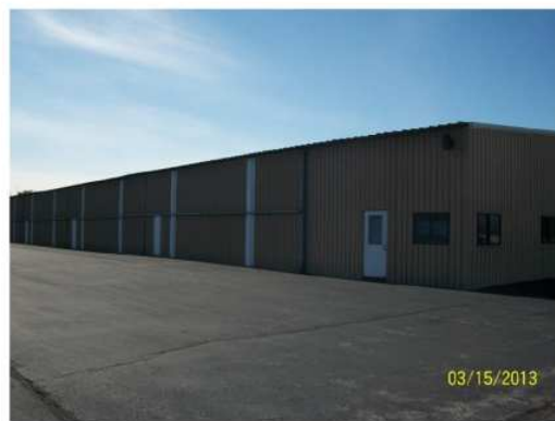
Figure 3: Overall view, Hangar A
