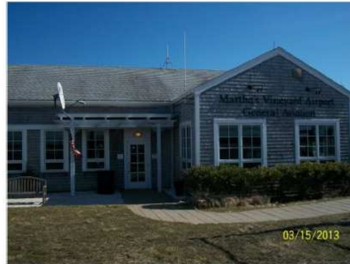
Figure 4: Airside View of Terminal
