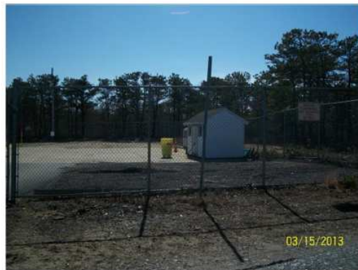
Figure 2: View of Fuel Farm Structure
