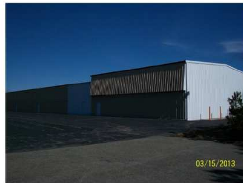
Figure 2: Front View of Hangar C
